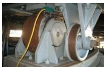
Simpson Avenue Bridge, a double-leaf Strauss trunnion bascule bridge, underwent a major rehabilitation including rehabilitation of counterweight trunnion machinery, span drive machinery span lock machinery, live load supports, and electrical power and control systems. WJE provided full-time on-site inspection of the mechanical and electrical work during critical closure periods and inspected manufactured components at the point of manufacture.
