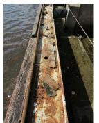
We performed an evaluation of the existing steel coating systems and conducted nondestructive thickness measurements of steel components to identify the severity of corrosion. Drilled core samples and steel coupon samples were obtained for laboratory testing.
