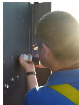
WJE evaluated the conditions of the coatings to identify possible approaches for surface preparation, recoating of the steel exterior elements. WJE also completed a thermal performance evaluation of the existing curtain wall. A series of trial repairs were tested through the installation of mock-ups of overcoating samples. The trials will then be reassessed after winter thermal cycling.
