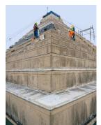
WJE developed construction documents to replace the roofing systems and remove all limestone cladding at the ziggurat, incorporate a new waterproofing membrane below the cladding, and install new lead-coated copper flashings.
