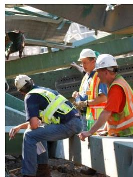
WJE engineers inspected all tension members for evidence of fatigue cracking and removed concrete cores from the deck and piers to determine concrete properties and deck weights. The engineers developed a detailed finite element model of truss connection to evaluate possible failure scenarios but ultimately determined that the failure was precipitated by the failure of gusset plates connecting the web members to the chord members at one of the nodes of the deck truss.
