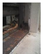
WJE made several inspection openings to confirm the components of the floor system and performed a structural analysis of the existing clay tile arch floor system and steel framing.
