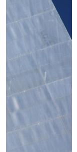
Observing increasing discoloration, streaking, and surface irregularity of the stainless steel exterior, as well as interior corrosion, the National Park Service sought an expert assessment of the structure to determine the source of the apparent corrosion and staining of the stainless steel; establish repair recommendations based on the structure's historical context; and develop a plan for long-term, sustainable protection.
