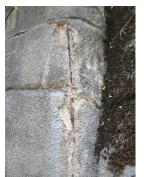
Given the age and weather exposure of the gunite themework, the walls were generally in fair condition with localized areas of significant distress. WJE provided conceptual repair options (along with corresponding advantages and disadvantages) for localized repair of the themework or over-coating the existing themework with a new, reinforced layer of qunite.
