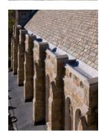
WJE's repair design and construction phase services included repointing of the stone facade, replacing perimeter seals around the windows, new lead-coated copper built-in gutters, and slate roofing repairs at the sanctuary and bell tower. The Church received the Restoration of a Sacred Landmark Award from the Cleveland Restoration Society and AIA Cleveland in May 2015.
