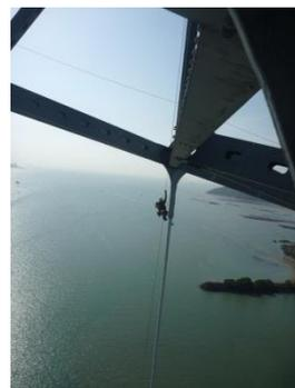
Areas within the bridge that exhibited distress or deterioration—primarily due to corrosion, fatigue cracking and initial concrete shrinkage—were examined in depth and the findings incorporated into the planned rehabilitation of the bridge.
