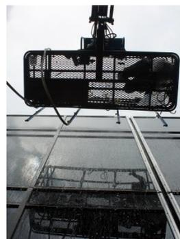
Extensive testing of the enclosure was performed, particularly at the glazing assemblies, to evaluate air and water infiltration resistance. The replacement cladding systems addressed by WJE as part of this project included a multi-layered metal panel wall assembly and a high-performance, multi-story, triple-glazed glass and aluminum curtain wall system.
