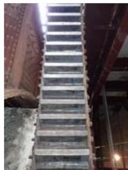
Structural and mechanical repair design was completed. Construction period services were then performed to assist the contractor in completion of rack tooth welded repairs to restore the existing teeth to their original profile, partial demolition and retrofit of existing machinery frame foundations, positioning of a new northwest machinery frame to provide optimal alignment/mesh with the repaired northwest rack teeth, and partial demolition and retrofit of existing leaf counterweight box.
