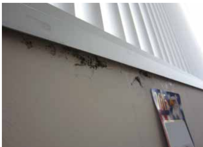
Typical thermal problems with existing window and wall systems include condensation and mold growth on interior finishes (left), as well as ice buildup on window frames and glass (right).
