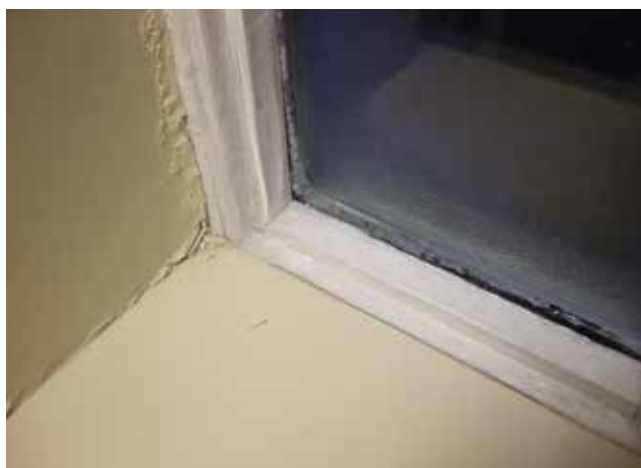
Typical thermal problems with existing window and wall systems include condensation and mold growth on interior finishes (left), as well as ice buildup on window frames and glass (right).
