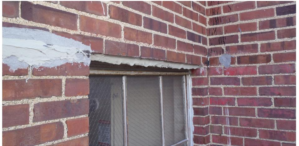
*Sealant improperly applied over flashing at the lintel spanning over a window opening*
