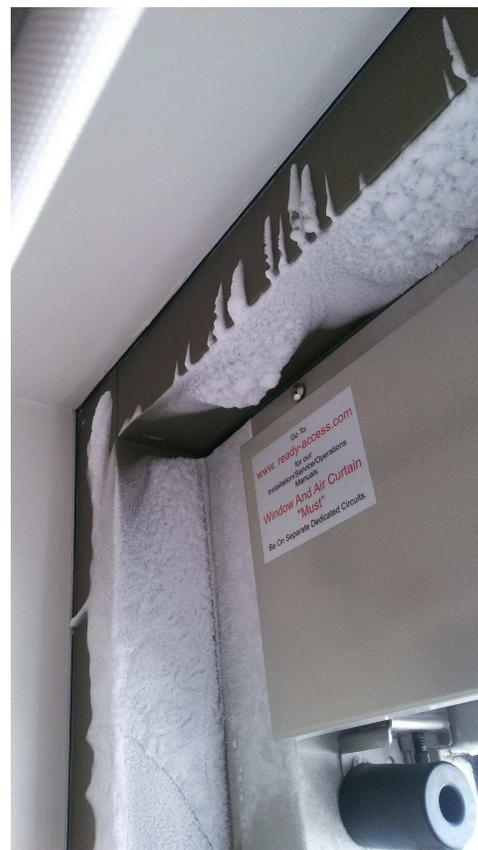
Severe frost/ice development on cold window frames due to condensation and thermal bridging issues (not a leak!)
