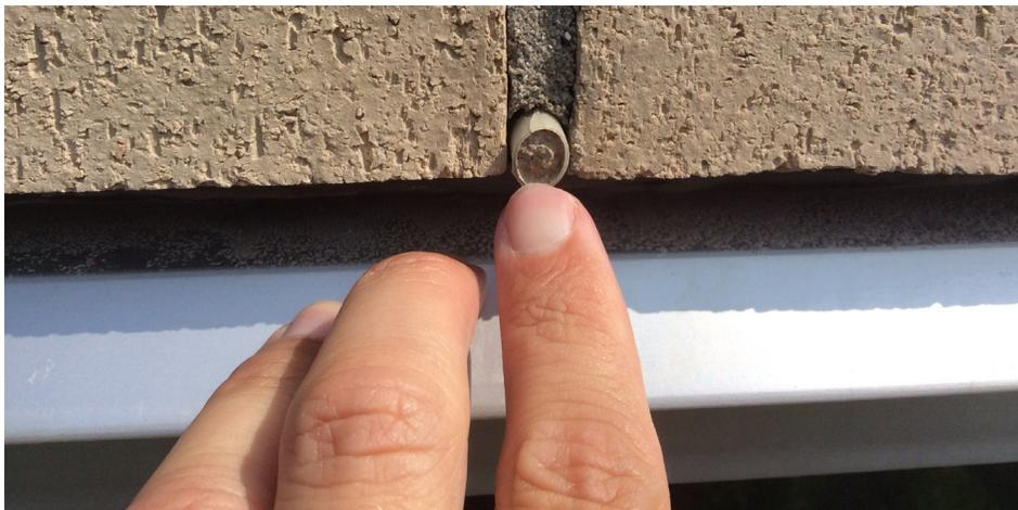
*Small plastic weep tube in masonry wall assembly above a window opening*
