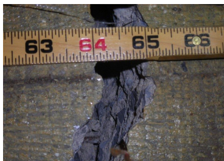
FIGURE 6. A ONE INCH-WIDE CRACK WITH A THREE-QUARTER-INCH VERTICAL OFFSET WAS DOCUMENTED IN A CONCRETE FLOOR SLAB OVER PYRITIC SHALE FILL. PORTIONS OF THE SLAB HAD HEAVED UPWARD MORE THAN TWO INCHES OVER THREE YEARS BEFORE THE SLAB AND UNDERLYING FILL WERE REMOVED.
