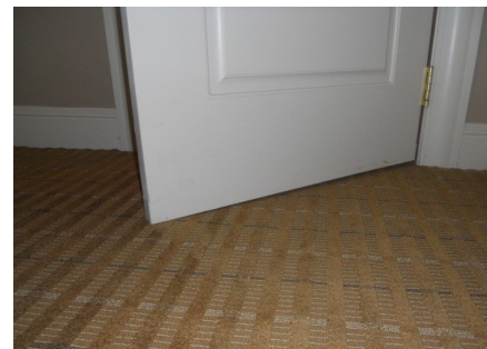
FIGURE 5. A HEAVED FLOOR SLAB HAS RESULTED IN A DOOR THAT CANNOT FULLY OPEN.
