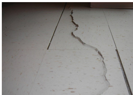
FIGURE 7. A FLOOR SLAB OVER PYRITIC SHALE FILL AND DOWELED INTO A PERIMETER GRADE BEAM EXHIBITED A LARGE CRACK WITH VERTICAL OFFSET AND ROTATION ABOUT THE DOWEL POINT INTO THE GRADE BEAM.
