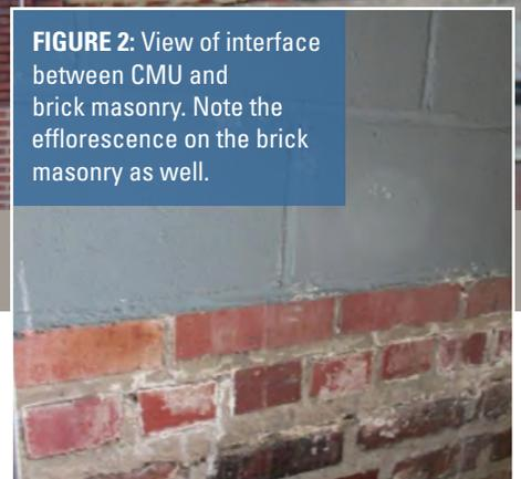
**FIGURE 2:** View of interface between CMU and brick masonry. Note the efflorescence on the brick masonry as well.
