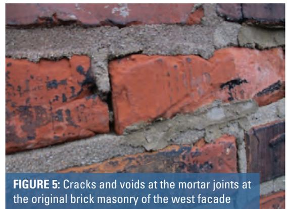
FIGURE 5: Cracks and voids at the mortar joints at the original brick masonry of the west facade
