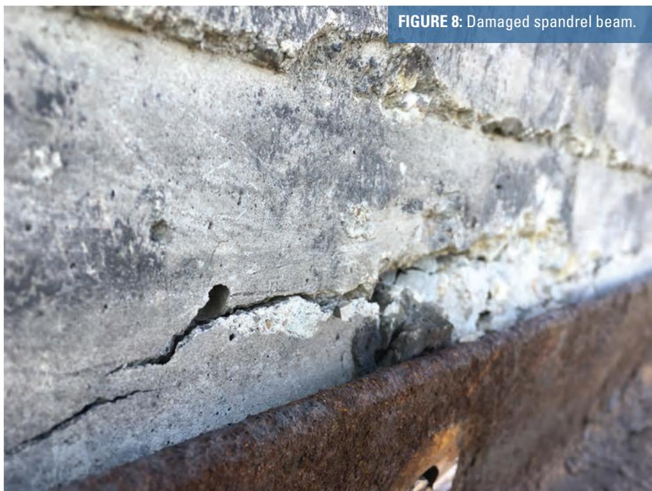
FIGURE 8: Damaged spandrel beam.
