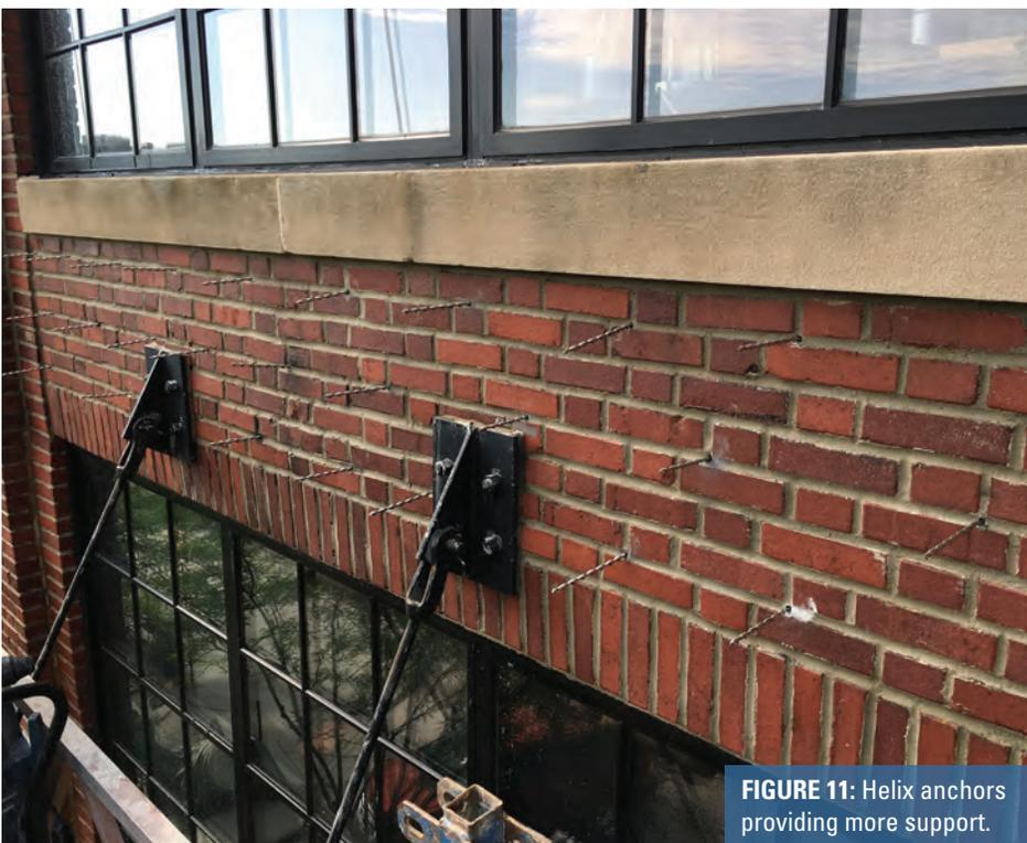
**FIGURE 11:** Helix anchors providing more support.
