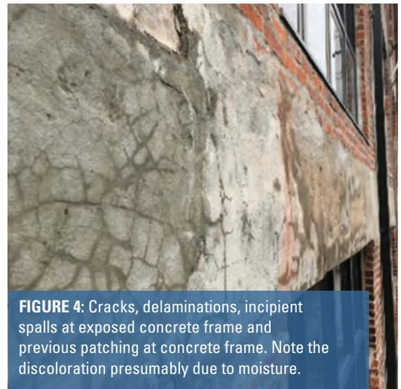
FIGURE 4: Cracks, delaminations, incipient spalls at exposed concrete frame and previous patching at concrete frame. Note the discoloration presumably due to moisture.
