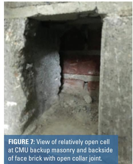
FIGURE 7: View of relatively open cell at CMU backup masonry and backside of face brick with open collar joint.
