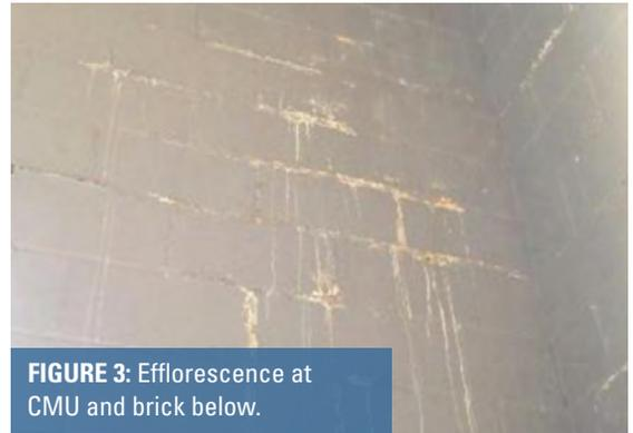
FIGURE 3: Efflorescence at CMU and brick below.
