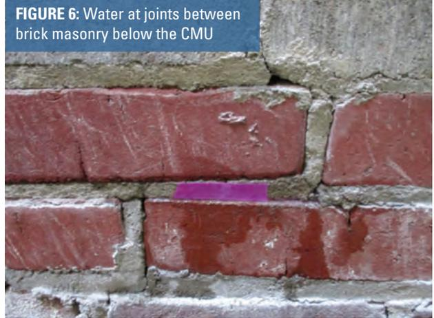
FIGURE 6: Water at joints between brick masonry below the CMU
