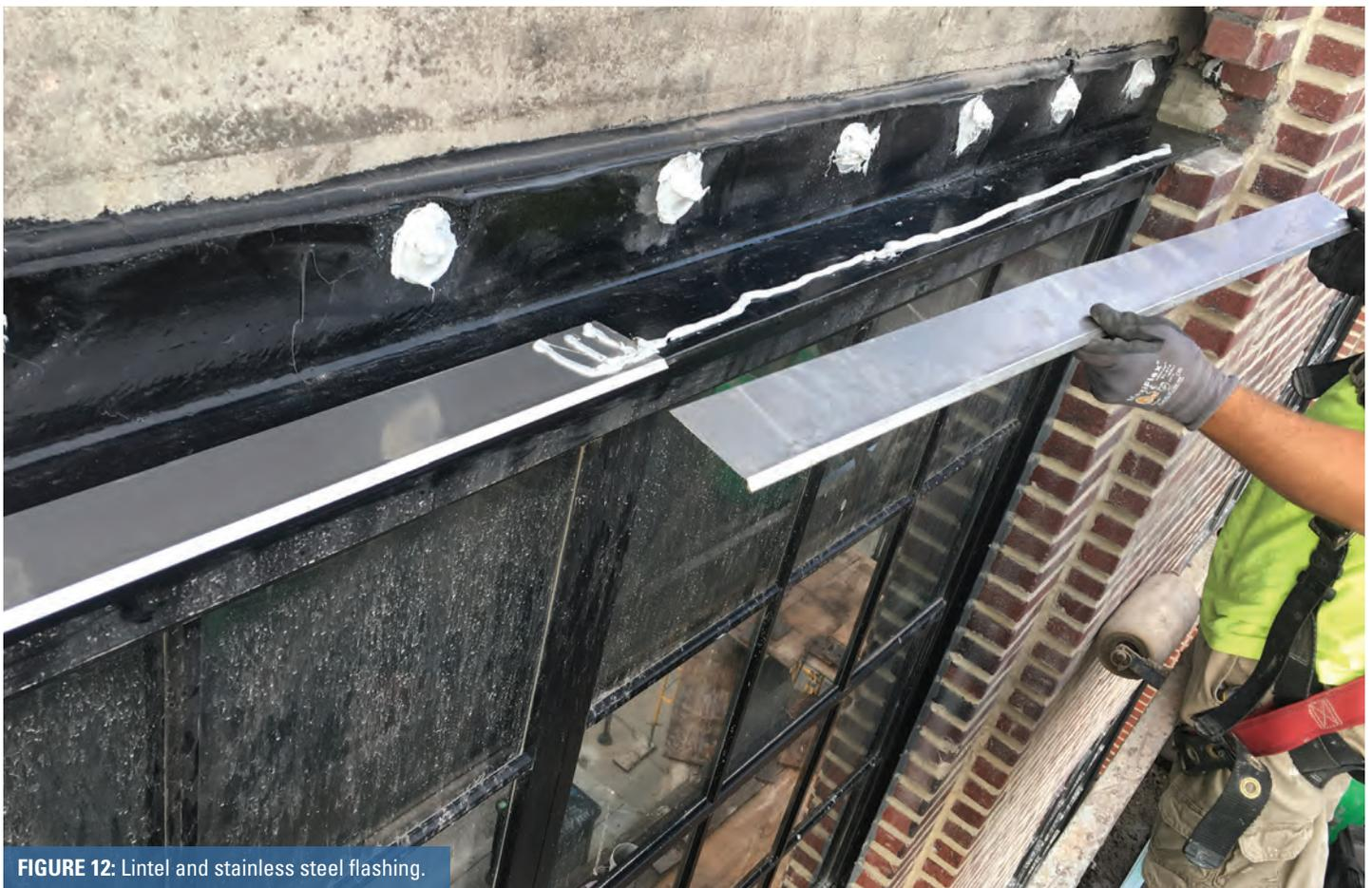
FIGURE 12: Lintel and stainless steel flashing.
