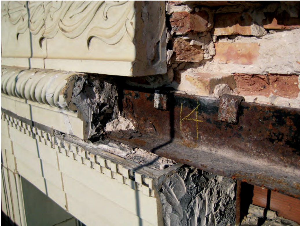
Fig. 6. New York Life Building, Chicago, 1889, terra-cotta lintel installation, 2013.
