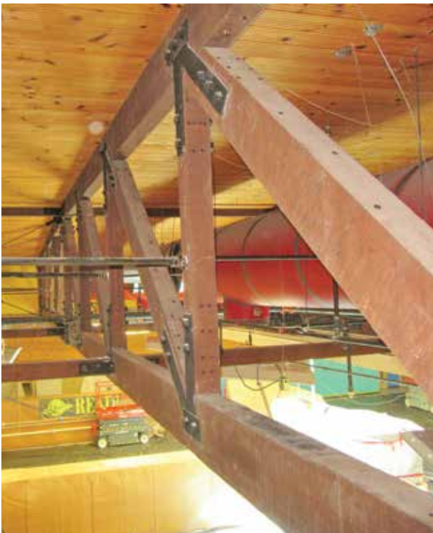
Repaired truss.
