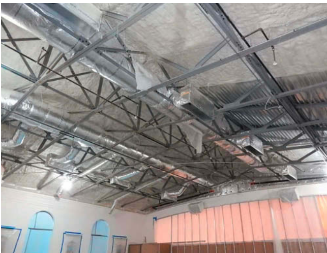
SPF Installation partially completed.
