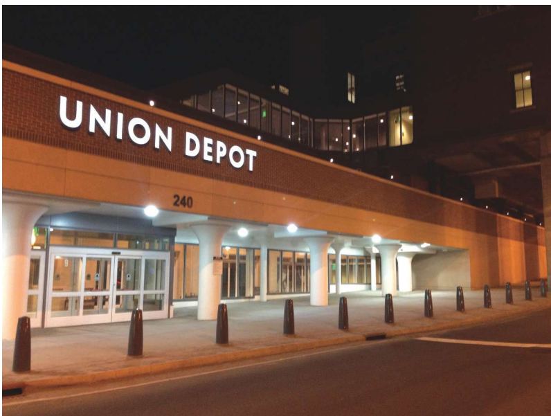
Fig. 9: Rehabilitated Depot entrance
