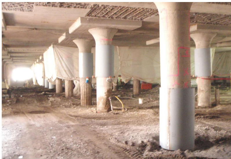
Fig. 6: Repairs in progress
