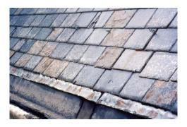
bothered to check the slate above, which had been removed, salvaged, and reinstalled to permit the gutter replacement work.
