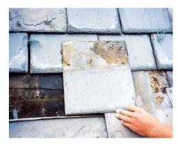
That's no optical illusion; the exposures of the slates in the fourth course above the copper gusset in the photo below taper from left to right. They should not taper. The result is minimal to no headlap at the far left end.
