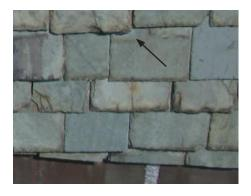
Photo to right: These slates were reinstalled with a two-inch offset. This places the nail holes in the slates below too close to the bond lines (joint between slate shingles). The nail holes, thus, become susceptible to water infiltration during heavy or wind-blown rains.
