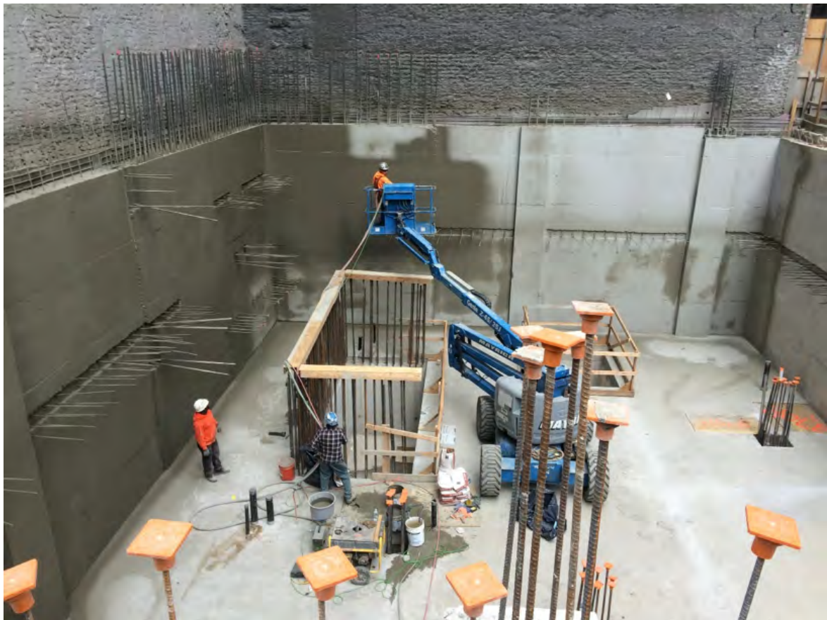
Application of crystalline, cement-based negative-side waterproofing.
