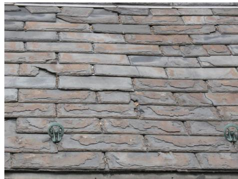
The Pennsylvania Black slate on the roof pictured at the top of the next column was installed c.1968. The roof contains a distinct pitch break, demarcated by the arrow. Slate on the upper section of the roof, where the slope is 13:12 (47°), is in decidedly better condition than that on the lower section of the roof, where the slope is just 6:12 (27°).
