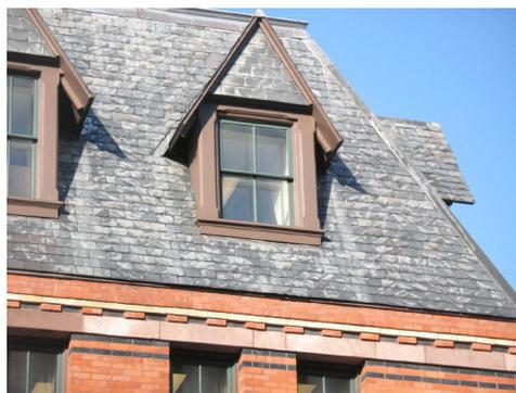
The final photo illustrates the condition of the slate on the 6:12-slope section of the roof. It is severely delaminated and contains many cracked and broken slates. It should be replaced now (or perhaps five years ago), whereas the slate on the upper section of the roof has a remaining service life of approximately ten years. The slate on the 6:12 slope suffered a reduction in service life of approximately twenty percent.
