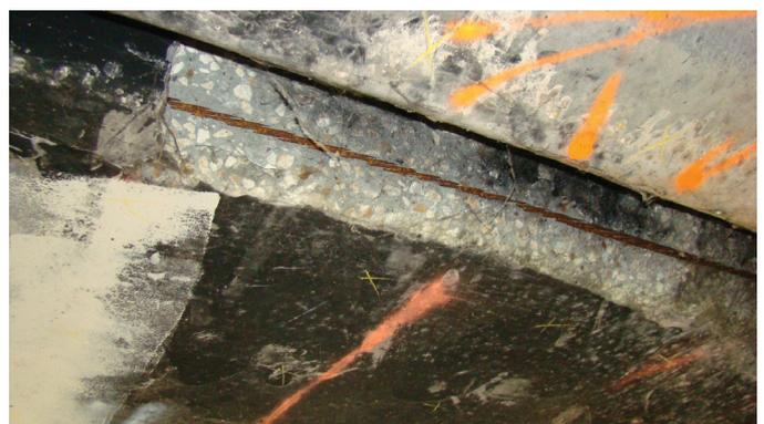
Fig. 4: Spalling of concrete box beam and exposed prestressed strand due to fire event
