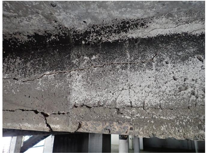
Fig. 2: Cracking along the length of a reinforced concrete joist due to fire exposure
