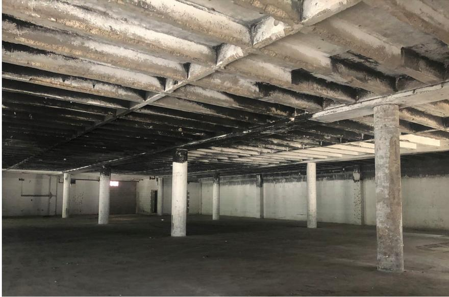
Fig. 1: A reinforced cast-in-place concrete structure that was damaged due to a fire event
