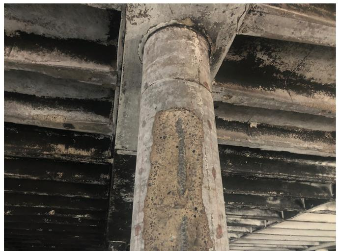
Fig. 3: Spalling that occurred on a concrete column due to fire exposure
