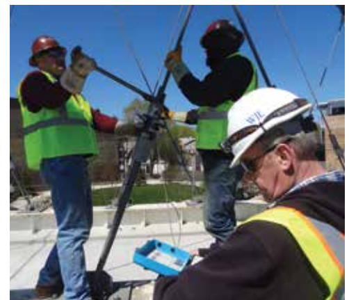
Figure 6. Tightening a cable and reading the load.
