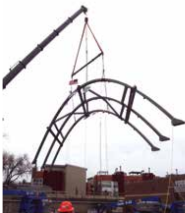
Figure 4. Lifting the arch assembly.
