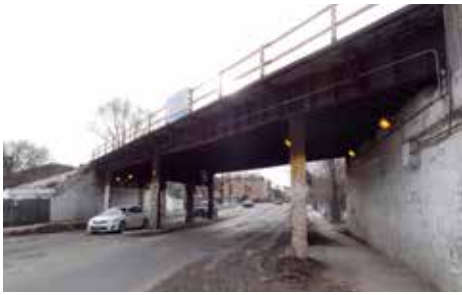
Figure 1. Existing bridge structure.
