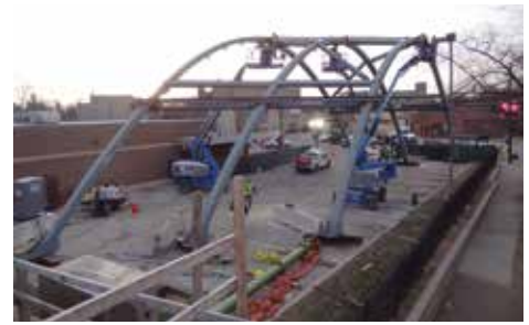
Figure 3. Erecting the three-arch assembly.
