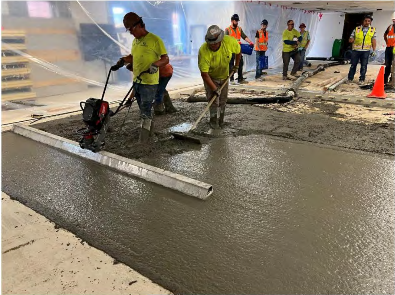
Figure 12. Representative photo of Slab 1 placement with Mix 1.
