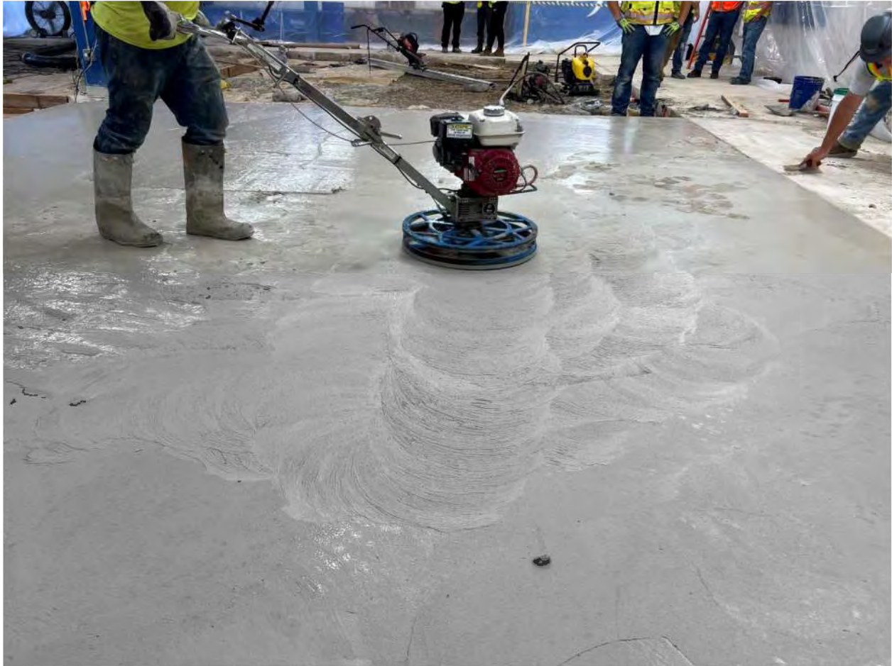
Figure 31. Slab 4, Mix 4 walkable pan finishing at edges.
