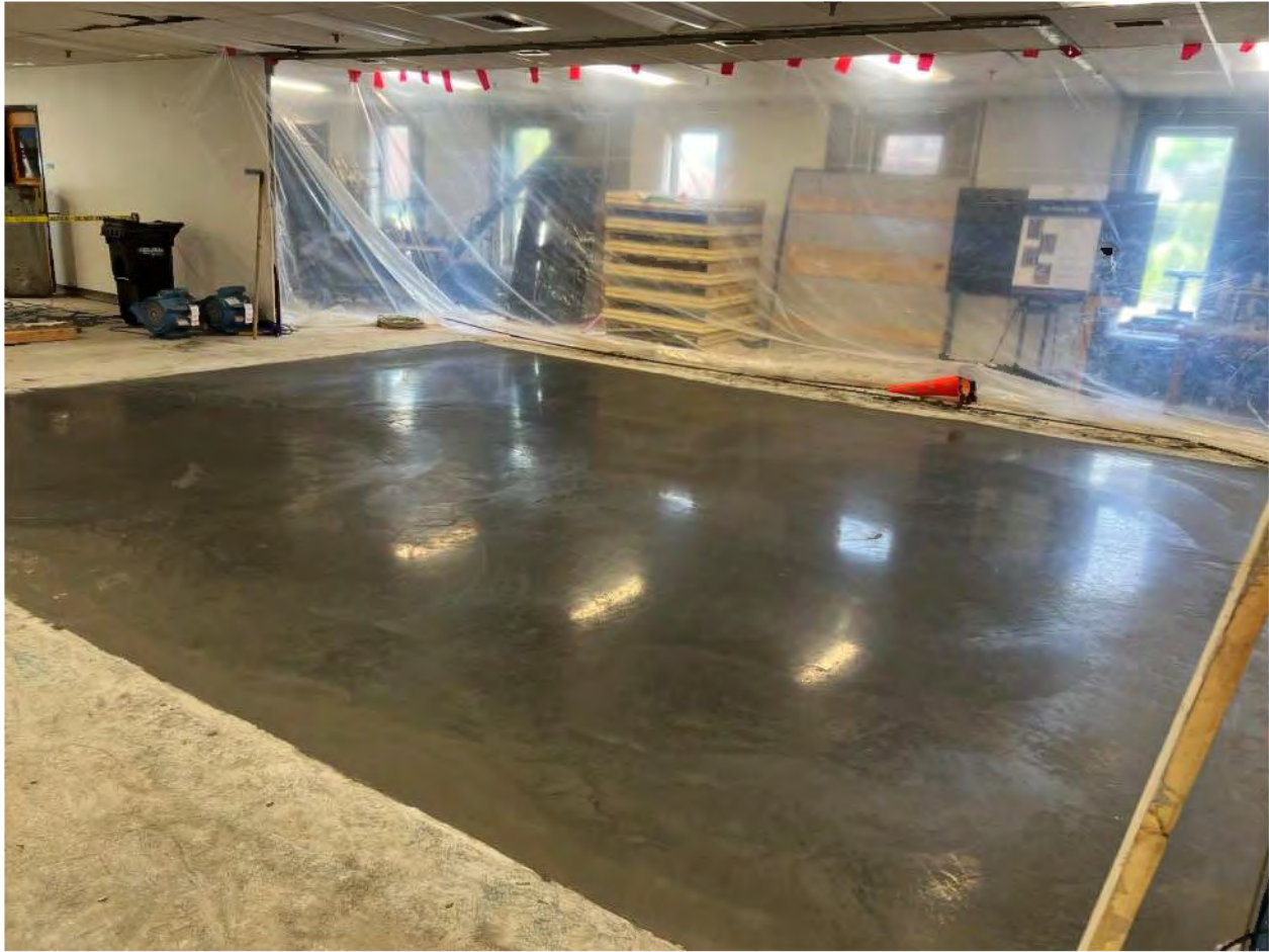
Figure 15. Slab 1, Mix 1 after completion of placement and power troweling.
