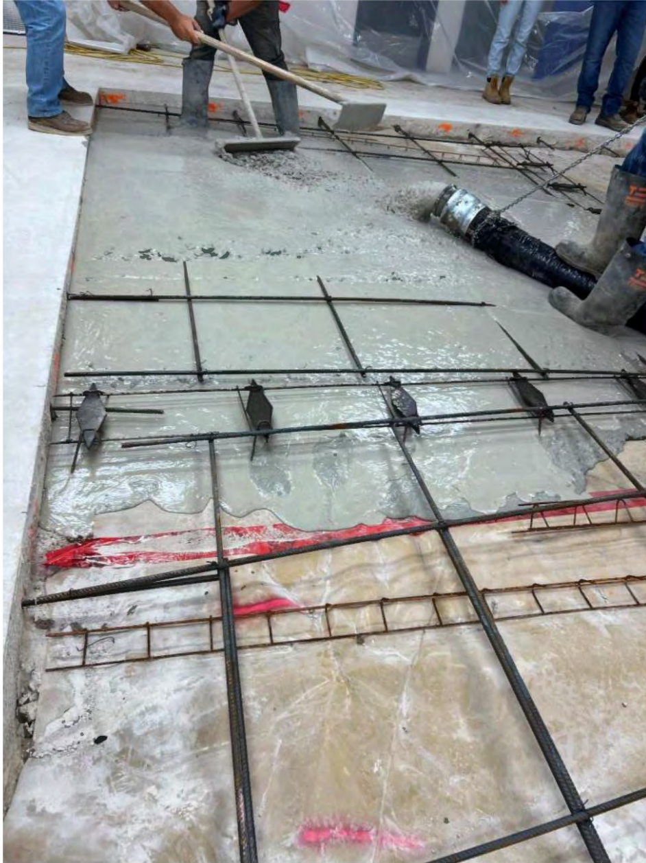
Figure 27. Representative photo of Slab 4, Mix 4 placement of Truck 1. Note aggregate and paste segregation.
