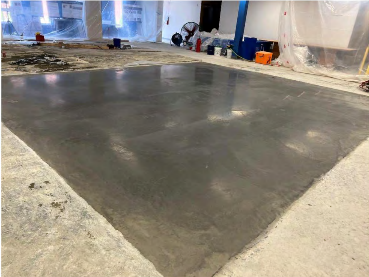
Figure 19. Slab 2, Mix 2 after completion of placement and power finishing.
