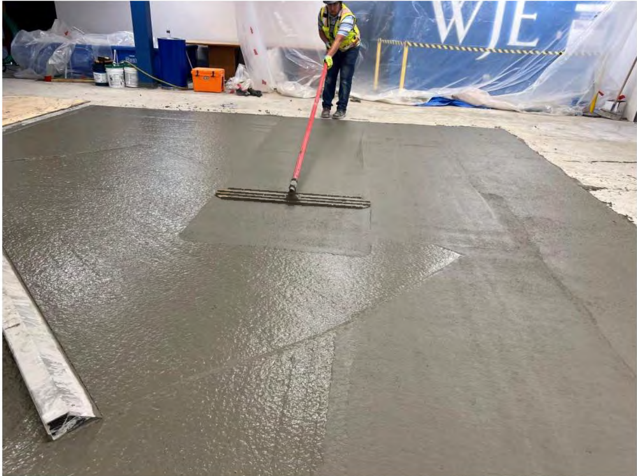
Figure 18. Slab 2, Mix 2 close-up photograph of concrete surface following bull floating. Note small amount of bleed water.
