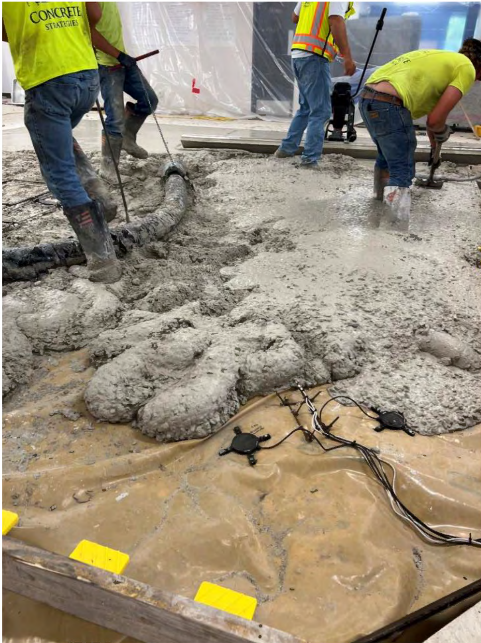
Figure 29. Slab 4, Mix 4 exhibiting thixotropic behavior in which the concrete sitting inside the pump hose from Truck 1 before arrival of Truck 2 became stiff.
