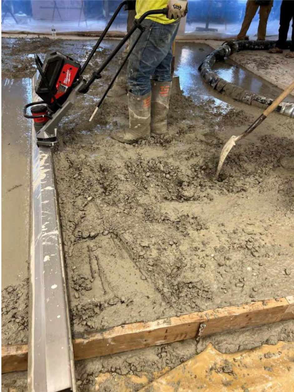
Figure 22. Slab 3 placement after Mix 3 became stiff and difficult to move.
