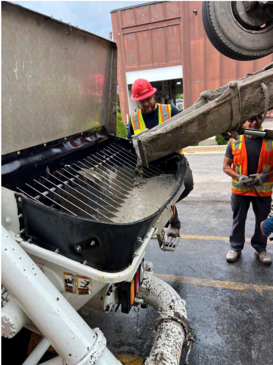
Figure 11. Mix 1, Truck #1 poured into hopper after Ozinga additions.
