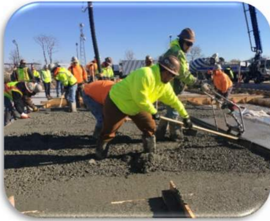
Figure 11. Vibratory screeding of Mix 1.
