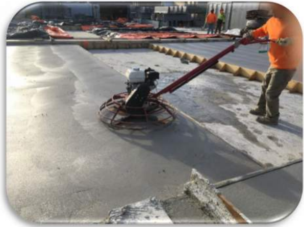
Figure 12. Light power trowel being applied to Mix 2.
