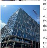
The two office buildings feature multiple waterproofed terraces and curtain wall system types. We consulted with the master architect team early on regarding the incorporation of granite fins into the unitized curtain wall system on one of the buildings.
