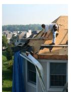
WJE observed the removal and repair of localized areas of roofing at forty leak locations on twenty-seven town homes and observed the complete roof replacement of three town homes at one building selected for roof replacement. Engineers also provided litigation support, including mediation hearing, preparation for jury trial, and deposition testimony in support of the association's successful claim against the developer and contractors.
