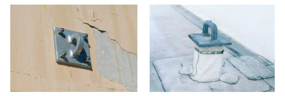
that they are capable of supporting 5,000 pounds in any direction for each employee attached. Certification by a qualified person, such as a professional engineer, is required at 10-year intervals (maximum). Many buildings that are less than 300 feet in height currently lack the tested, certified, dedicated anchorages required to use rope descent systems in compliance with OSHA regulations.
