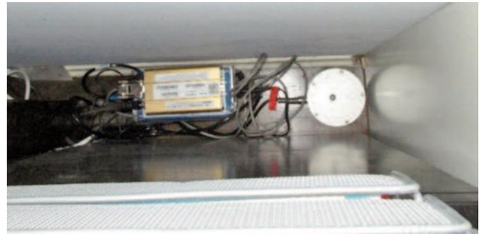
Figure 4. Looking down at typical vibration monitor installation.
