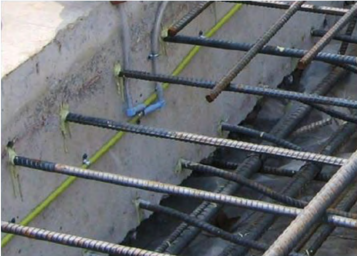
Injection grout tube at construction joint. PHOTO COURTESY OF GCP APPLIED TECHNOLOGIES
