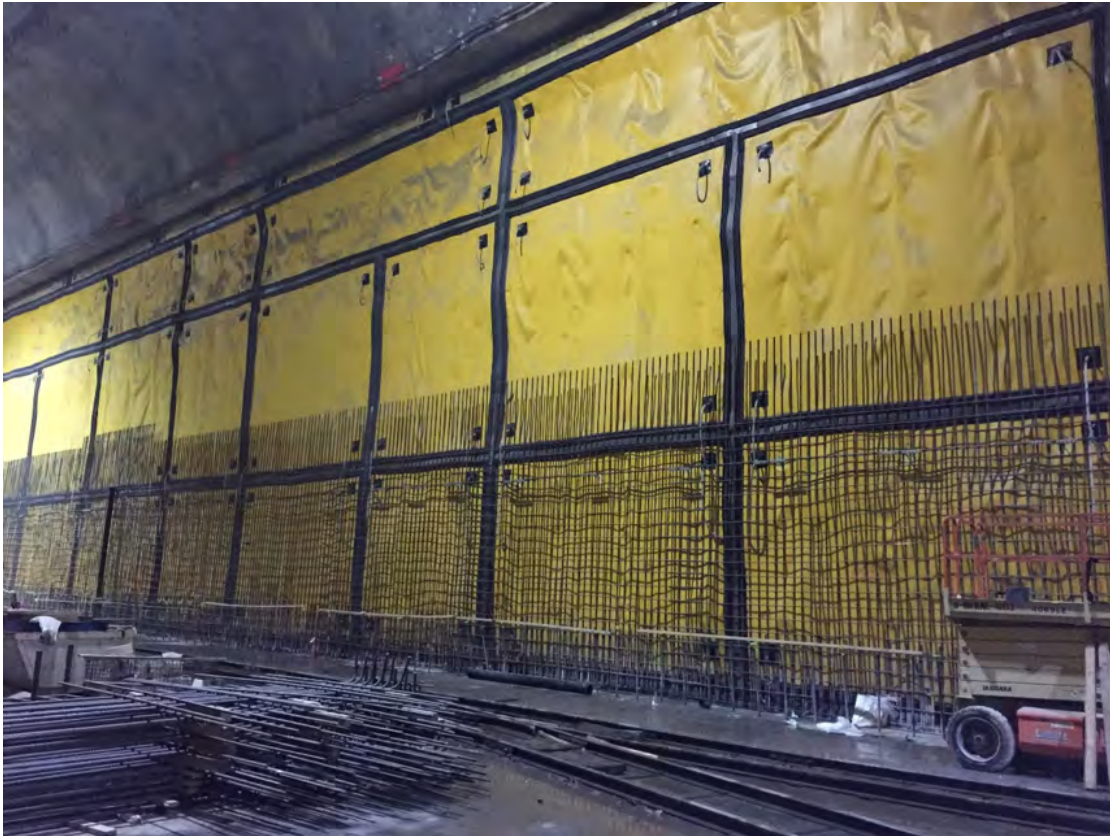
Blindside waterproofing membrane with integral compartmentalizing system and injection ports for grouting after concrete placement.
